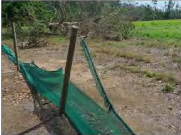
Figure 4.24 Cyclone Yasi 300m fence - south. Clip did not release and fence ripped
