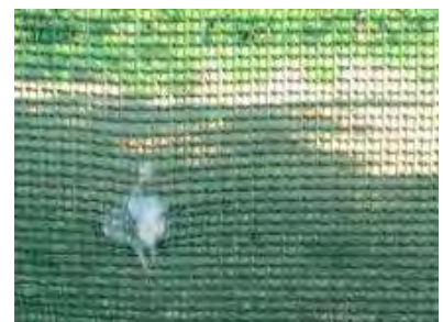
Figure 4.38 Temporary repair using silicone
