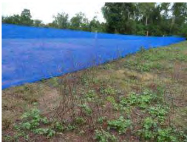
Figure 4.6 Trial #2 Fence completed
