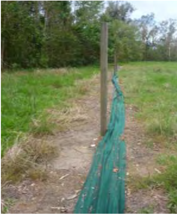
Figure 4.20 Cyclone Yasi 100m fence dropped and tied - no damage
