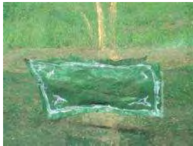
Figure 4.36 Temporary repair using glue on patch
