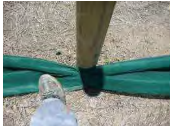
Figure 4.13 Contained fence to posts
