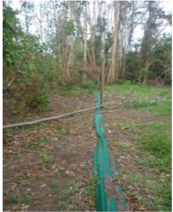
Figure 4.21 Cyclone Yasi 200m fence dropped and tied – no damage
