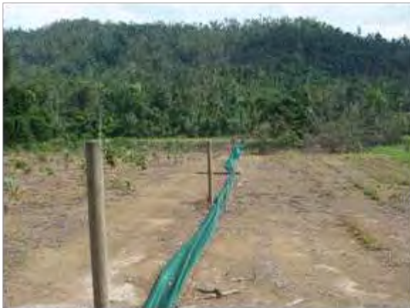
Figure 4.22 Cyclone Yasi 300m fence- south No damage to shade cloth locally
