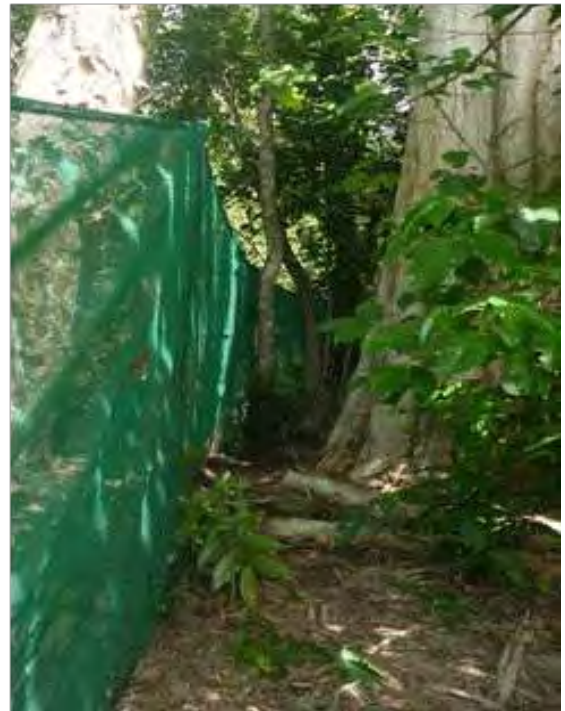
Figure 4.29 Cyclone Yasi 200m fence after re-clip showing minimal impact
