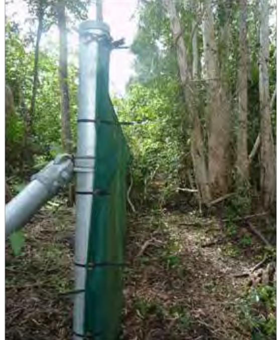
Figure 4.16 End View Fence through riparian vegetation Untouched for 1½ years
