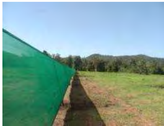
Figure 4.19 fence lay down from high wind
