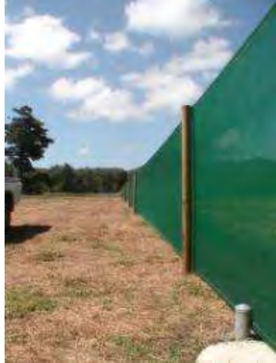
Figure 4.11 Fence erected for revegetation lot.
