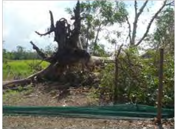
Figure 4.25 Cyclone Yasi 300m fence south. Tree up-rooted, no damage locally
