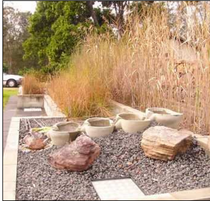
Figure 4: Example of a reed bed system to treat recycled water
