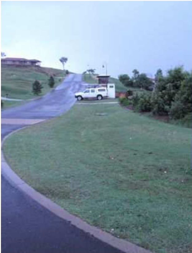
Figure 8: Example of a vegetated swale.
