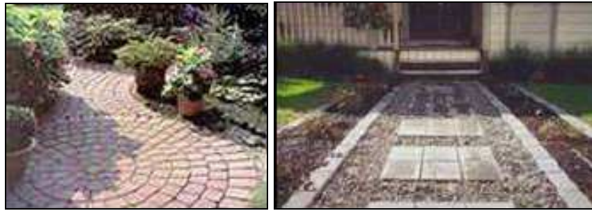
Figure 14: Examples of porous pavement
