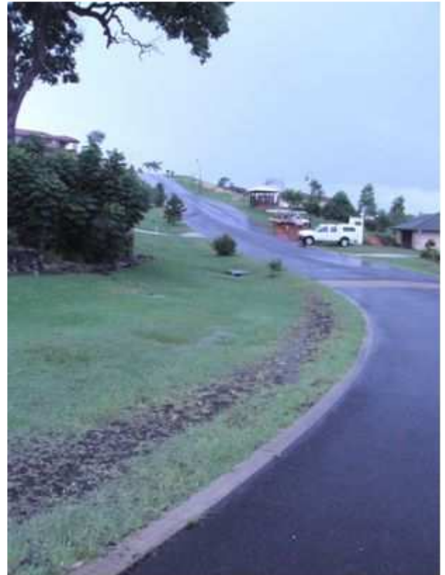
Figure 9: Example of a vegetated swale
