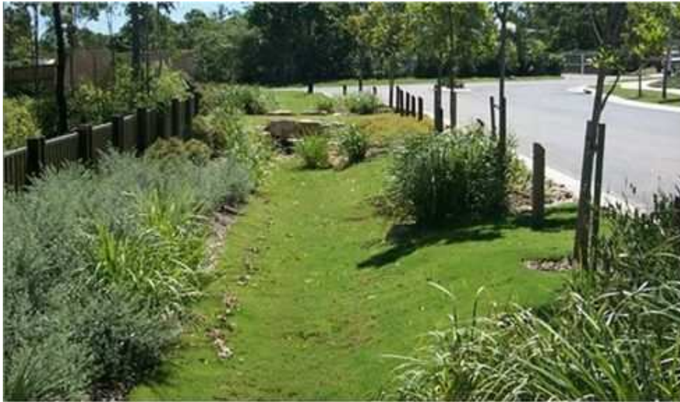
Figure 10: Example of a vegetated swale.
