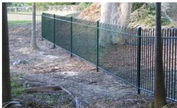
Figure 2:2 Aluminium loop style pool fence
