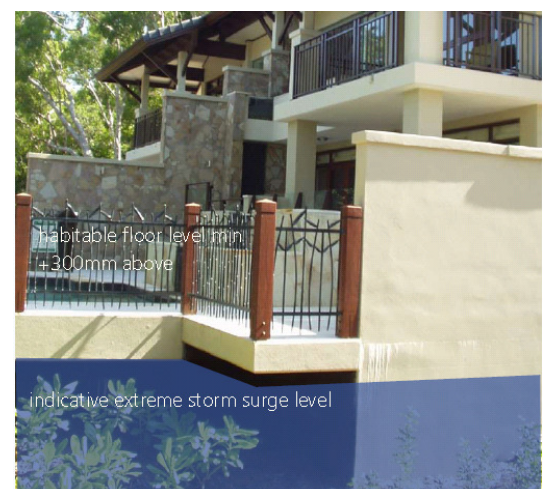
Figures 1.7.15–1.7.18: Construction techniques for potential flood/storm surge zones
