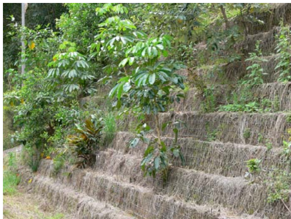
Plate 8. Fallon Road Terramesh units after 20 months (August 2007). Shows northern end where establishment has been very successful.
