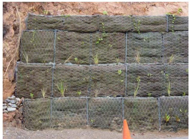
Plate 15. The wall under construction (March 2004).
