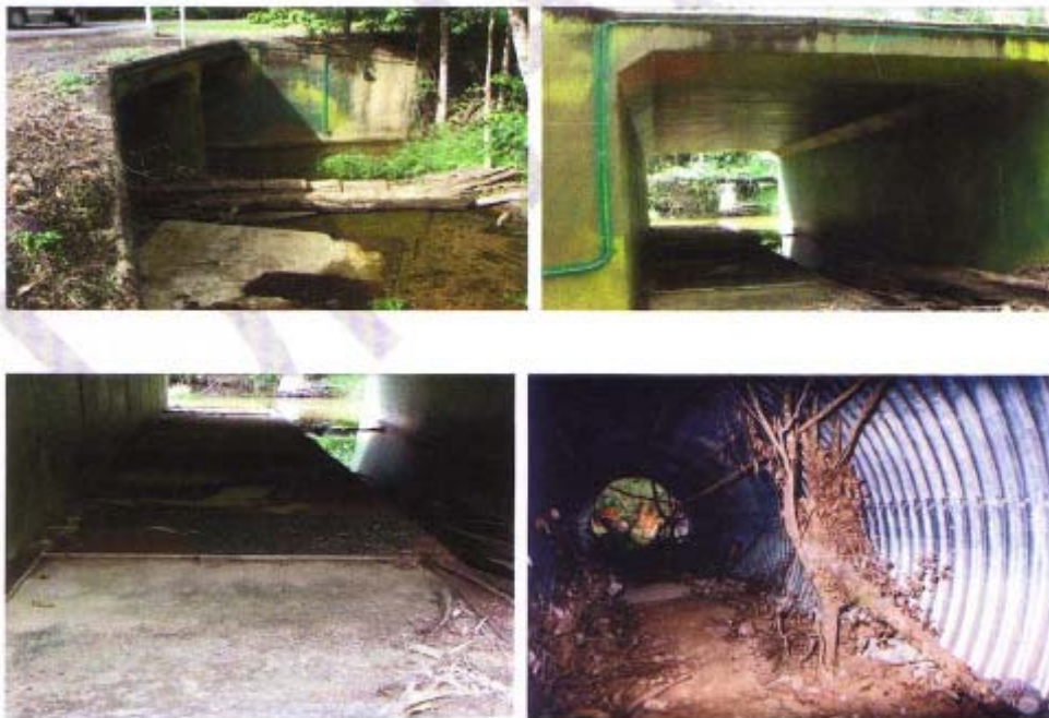
Figure 4-7: Faunal underpasses depicting 'furniture', including escape pole (vertical tree branch), dry ledge, sand bed, attractive habitat at exit, soil, litter, rocks and logs to simulate rain forest floor conditions (Biotropica; Goosem et. al. 2005)
