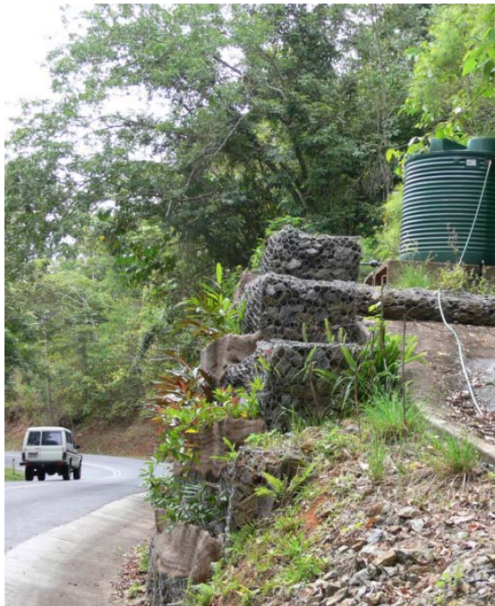
Plate 13. Sometimes a temporary water supply may be desirable as was the case for this example on the Kuranda Range Road (August 2007). In this case the tank could be filled by gravity from a nearby permanent stream.
