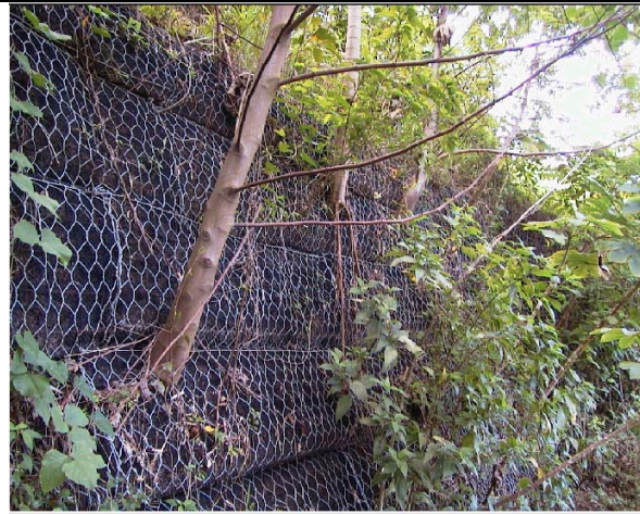
Plate 20. Large trees growing through Terramesh gabions (overseas project).
