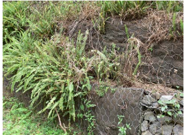
Plate 17. Close-up of section of lined gabion showing build-up of leaf litter on the gabion ledge and denser establishment of ferns.
