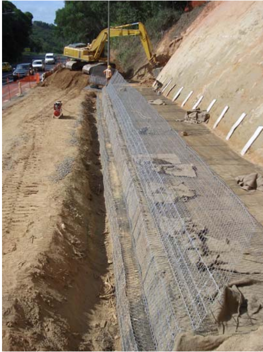
Plate 6. Installing Fallon Road Terramesh units (December 2005). Fallon Road is on the Kennedy Highway just west of Kuranda.
