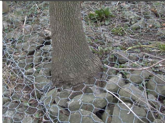
Plate 21. Close-up of a large tree growing through Terramesh gabions (overseas project). The mesh becomes integrated into the plant structure, apparently without causing weakness to either the plant or the gabions.
