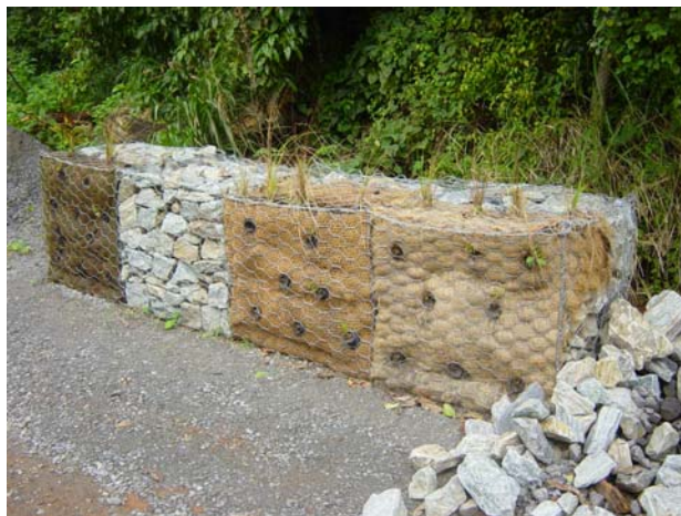
Plate 14. Gabion units during construction (March 2004).
