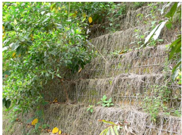
Plate 9. Fallon Road Terramesh (August 2007). Shows successful establishment of septic fig ( Ficus septica ).
