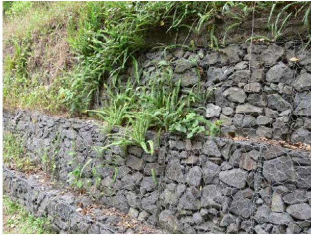
Plate 16. Close-up of section of unlined gabion showing establishment of ferns.
